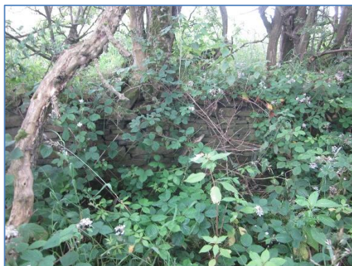
Figure 15: Overgrown Stone Wall at the East of the Site
